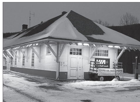
The Matapedia train station was built in 1903 and has received heritage status from both levels of government before 2000.
