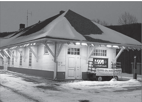
The Matapedia train station was built in 1903 and has received heritage status from both levels of government before 2000.
